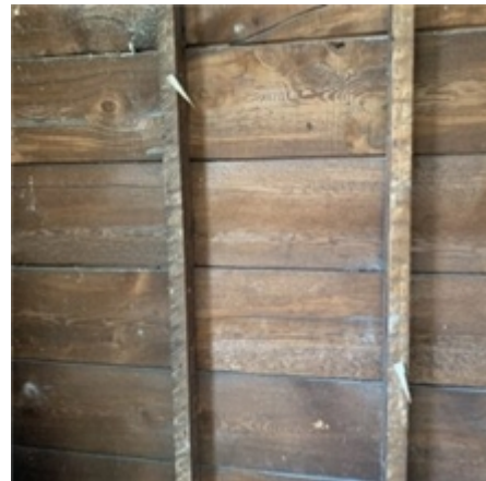
Sample image showing similar exposed wood framed wall
